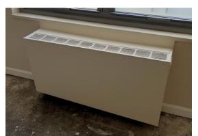
Air conditioning season is around the corner. Some shareholders encounter convector leaks due to condensate or dirt and/or debris build up in the convector trays, which result in blockage and cause water flowing through the convector trays to overflow onto their floor. To avoid this, please find a list of proper steps and procedure below to keep your convectors clean and free of debris and objects.
